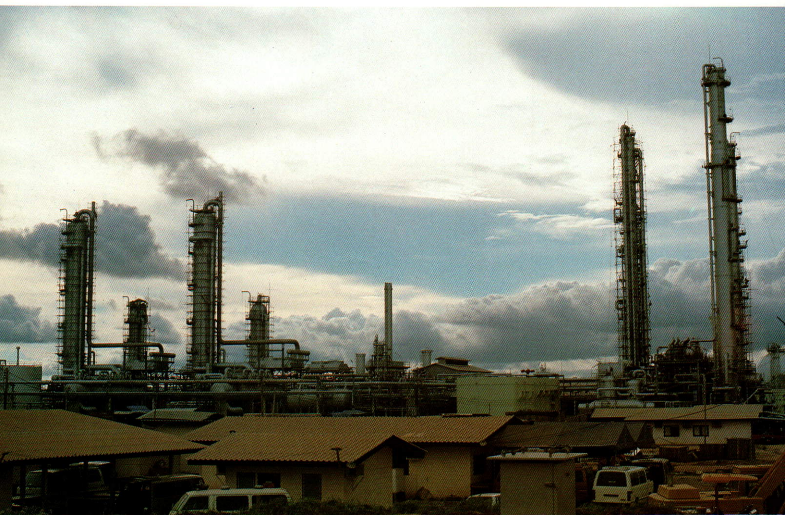
6. Gas Separation plant at Rayong Province designed for a total capacity of 350 MMSCFD of feed gas.
