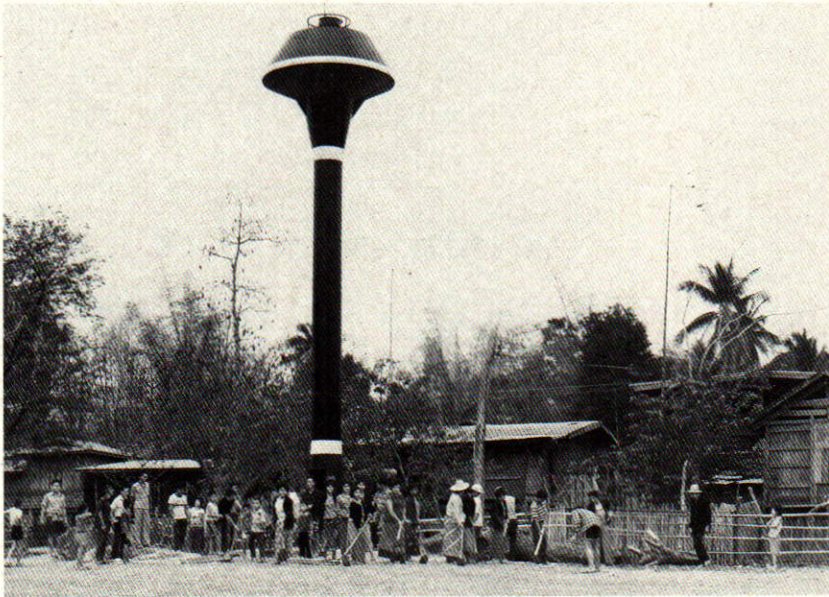
1. Ban Mou Mon Water Supply Project - funded in 1983 - a water tank was installed over an artesian well - Udon Thani Province.
