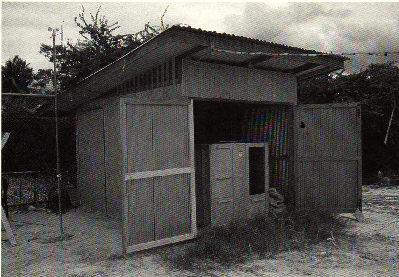
9. Forced Convection Solar Hut Dryer developed under U.S.-Thai Renewable Energy Co-operation Project. The solar hut dryer functions simultaneously as a dryer and a storage barn.
