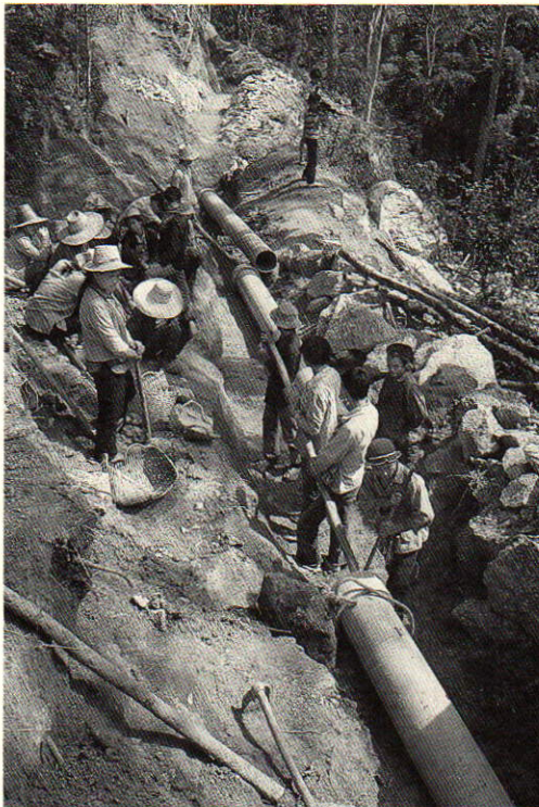
2. Headrace pipes were laid by villagers.
