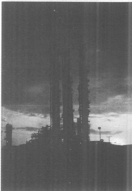
PETROLEUM AUTHORITY OF THAILAND GAS SEPERATION PLANT 1 UNDER CONSTRUCTION.
