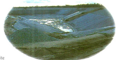
In-site reservoir under expansion to 5 million cu metre storage capacity with PVC lining.
