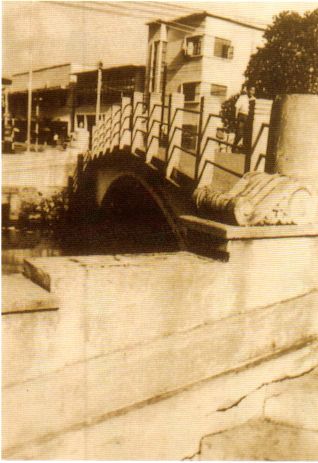
Bridge over Wat Anongkharam canal
