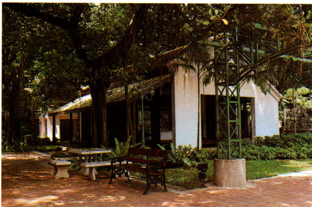
The replica of the house during construction
