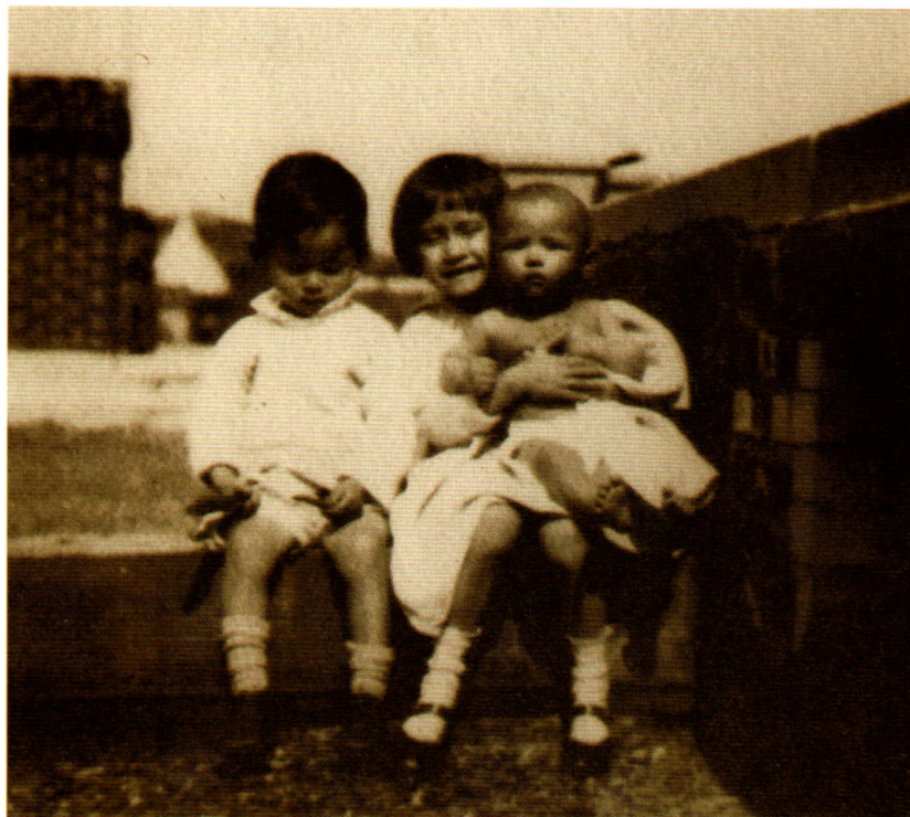
On the roof of the Boston home
