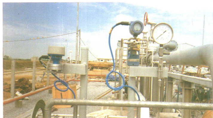
INSTALLATION OF INSTRUMENTATION
