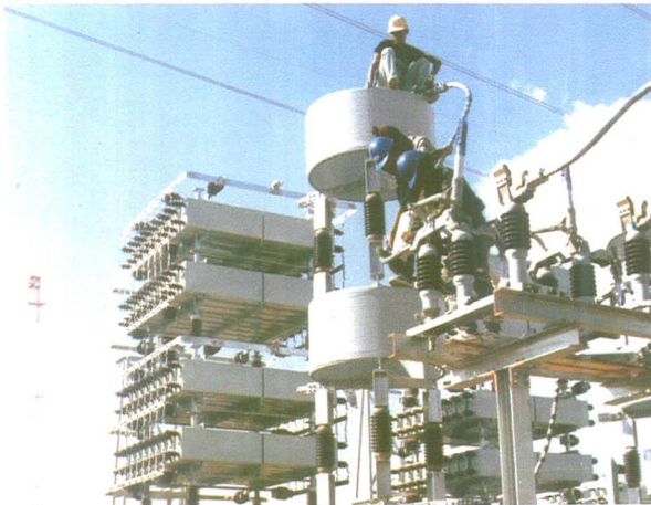
INSTALL ELECTRICAL EQUIPMENT 22 KV SUBSTATION
