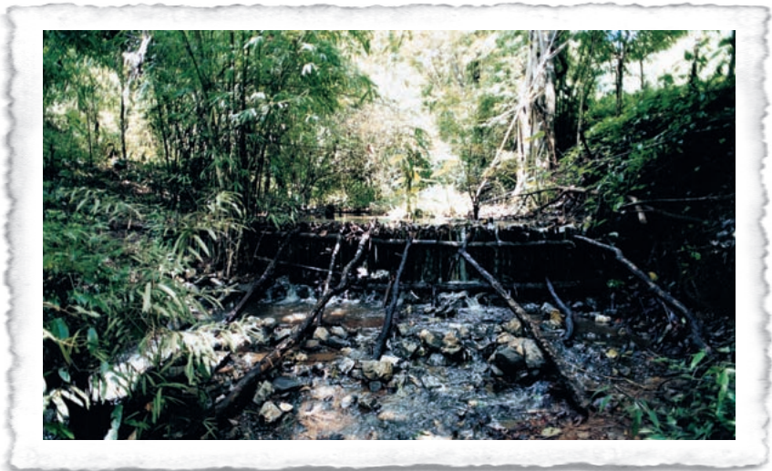
A check dam at Huai Hong Khrai, Chiang Mai Province.
