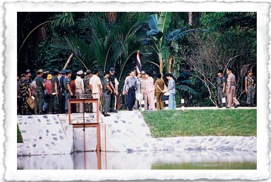
His Majesty views the impounding dam for irrigation purpose.
