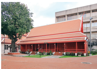
The Red Residence was built in King Rama II's era as his Queen's residence. Formerly, it was located inside the Grand Palace, before being moved to the National Museum Bangkok in the reign of King Pinklao, the second king in the reign of King Rama IV.
