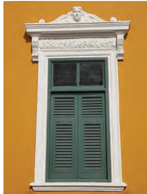
Phra Ratchawang Metro Police Station: Formerly a palace ground, the original construction was demolished in King Rama VI’s era and rebuilt as a police station in 1915, designed by Italian architect Mario Tamagno under the Department of Public Works. It is a one-story building with a load-bearing wall system and reinforced concrete structures, a new construction technique at the time.
